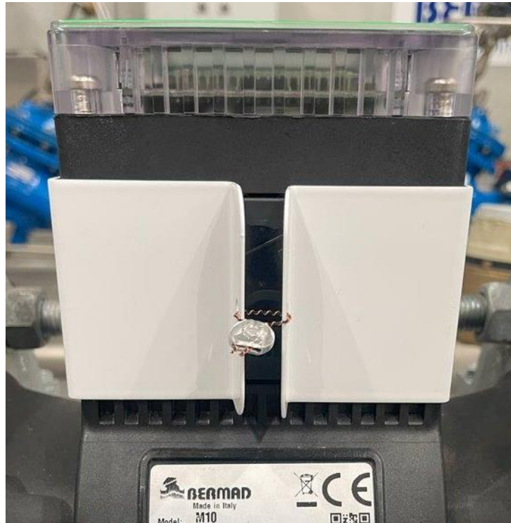
Bracket to facilitate sealing
